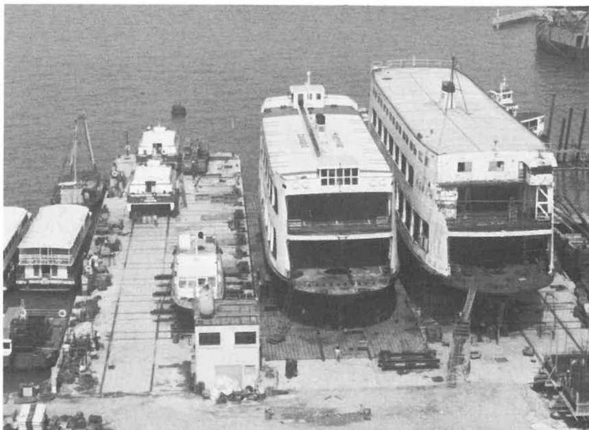
Hong Kong Shipyard Ltd is one of the two companies that use Syncrolift for docking repair.
